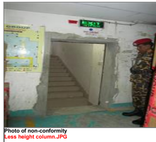
Photo of non-conformity Handrail not installed in both sides.JPG
