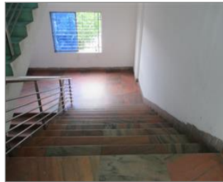
Photo of non-conformity Handrail not installed in both sides.JPG
