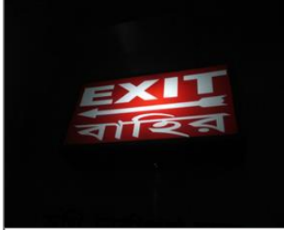
Photo of fire safety equipment Exit sign.JPG
