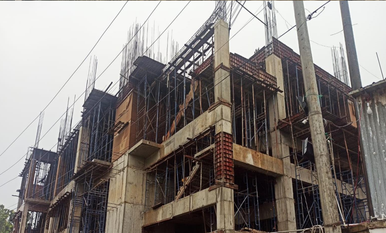
Present Condition (Work in Process)
